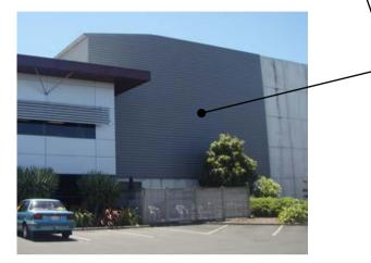
This large industry locates the office/administration component of its operation closest to the street at a lower height to the main plant area. A painted corrugated iron panel and concrete texturing has been used on the factory frontage. This relatively low cost design feature goes a long way to improving an otherwise very dominant blank concrete wall.
