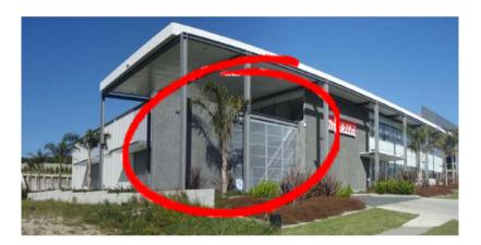
A false façade and gate provides for a very secure, safe, and screened servicing, loading/unloading, and storage/collection of wastes away from the street.
